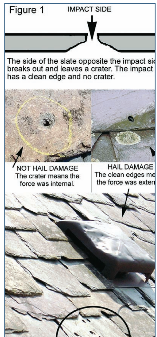
Figure 1 - When slate is perforated, the impact leaves a clean hole on the impact side and a cratered hole on the opposite side of the impact. (All photos by Joseph Jenkins.)
